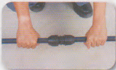
3. Masukkan pipa PE Blue Line kedalam fitting hingga batas akhir fitting.
